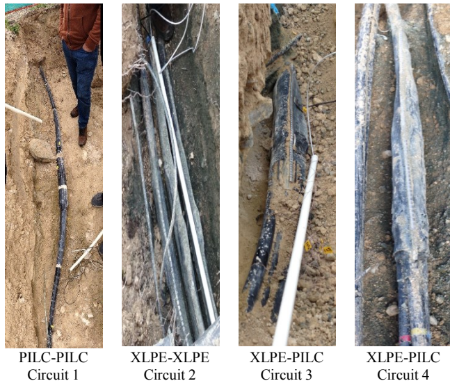
Fig. 1 Cable joints under investigation
